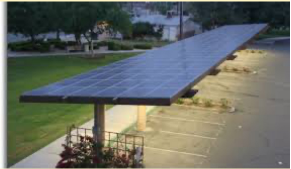
Example of a Carport Photovoltaic Structure
