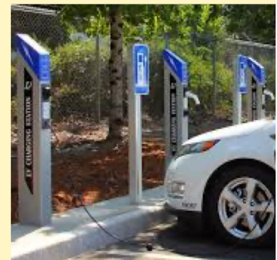
Example of a Vehicle Charging Station
